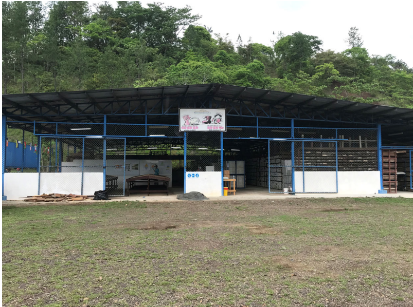
Figure 12.1 Core Storage Building (MMTS, 2021)
